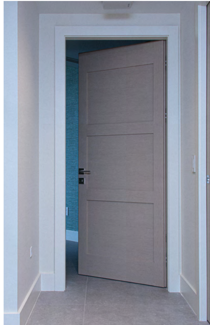
TELAIO/ doors with raised casing
