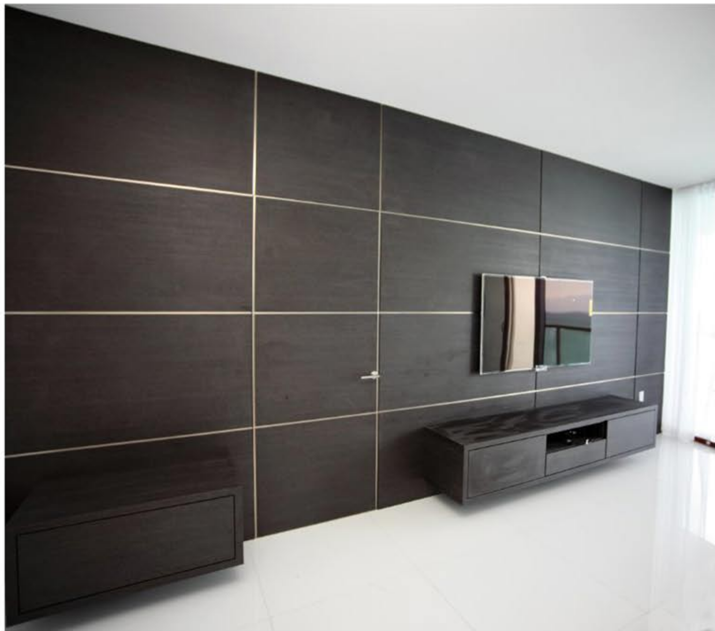
Panels/ Wenge with 1/2" stainless steel reveals and invisible door application
