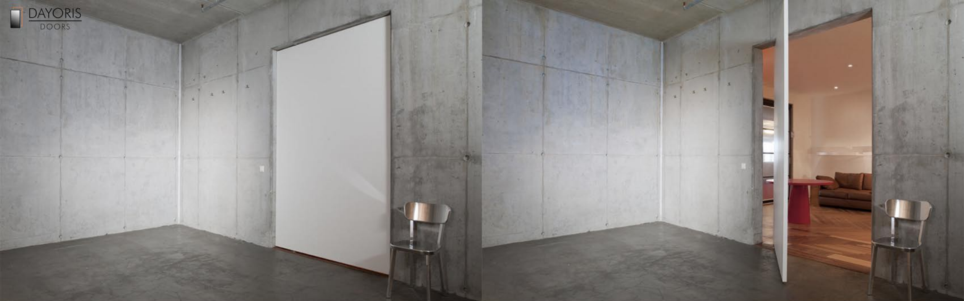
Filo Muro/ lacquer finish, pivot system
